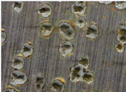
Microbiologically Influenced Corrosion
