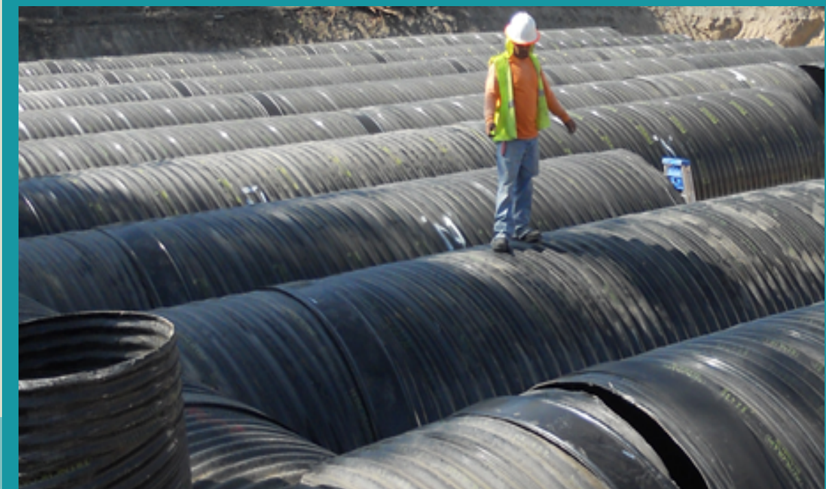
8' DIA. GIANT TUBES UNDER GREEN SPACE FOR RAINWATER STORAGE
